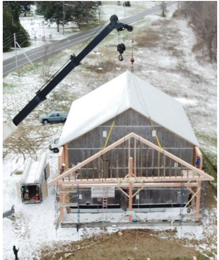
Construction in progress at the Farmington Quaker Meeting House.
